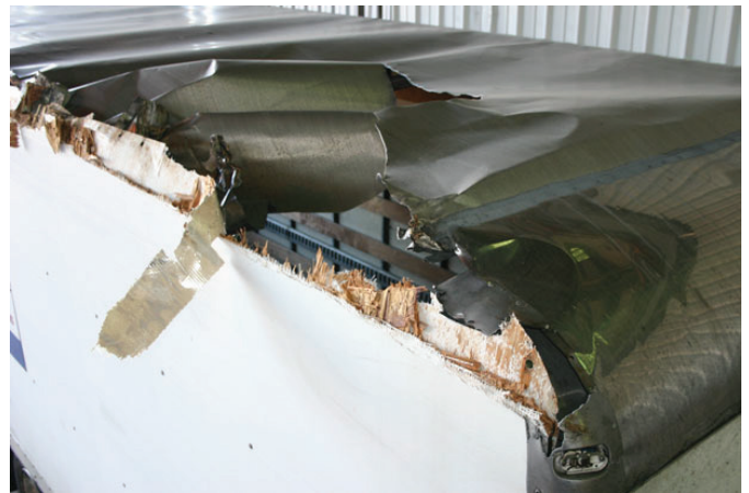
Roof Repair & Replacement
