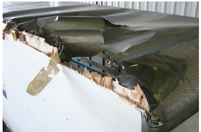
Roof Repair & Replacement
